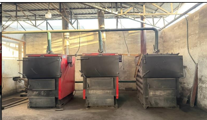
Example of Biomass Pellet Vacuum Boilers Provide Heating for the Building in winter
