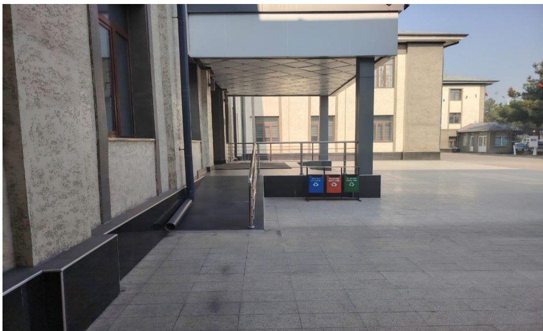
2.7-ramp Administrative building
