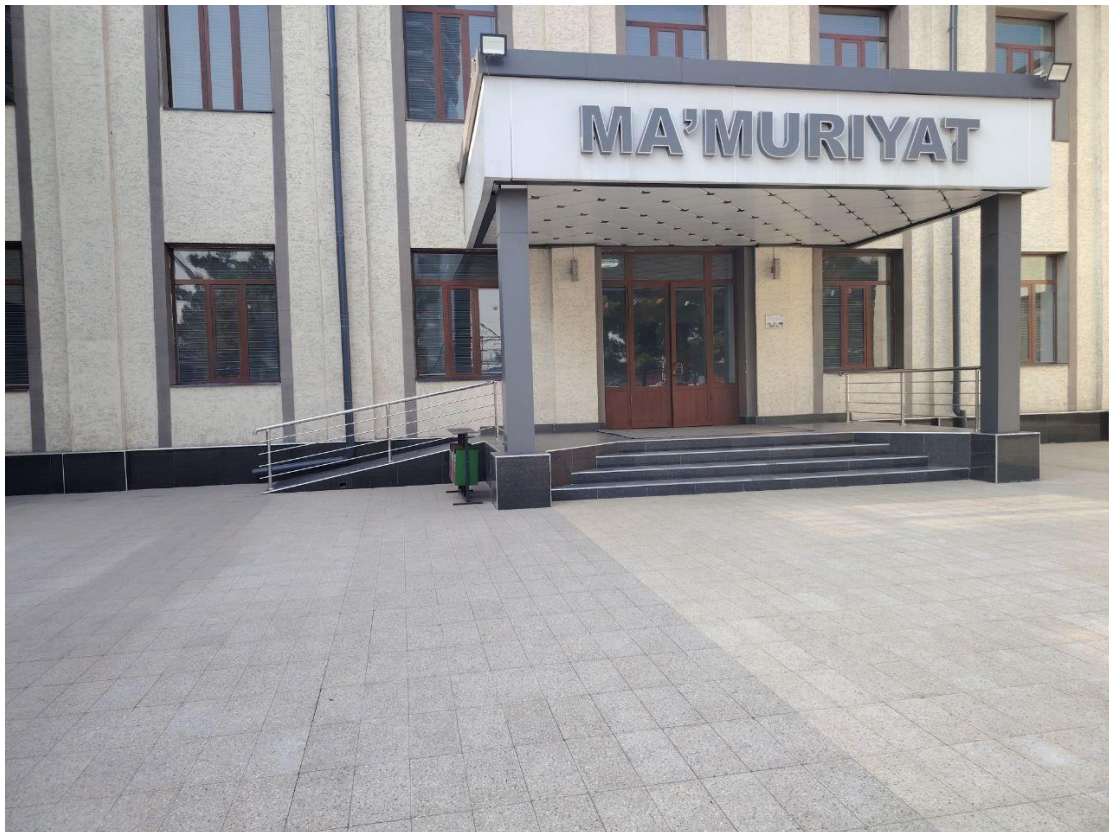
2.8 Ramp Administrative building
